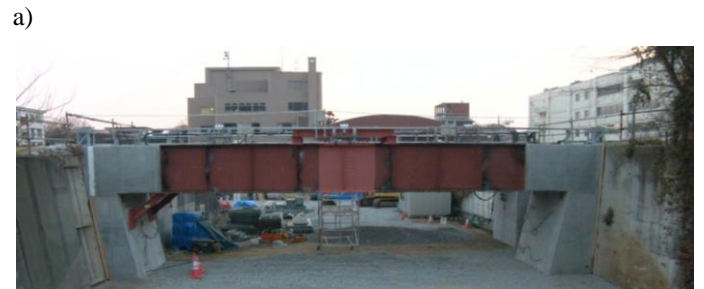
Figure 42. Full-scale model of conventional type bridge reinforced by nailing of the backfill and integrating the girder to the abutments; a) overall structure; and b) a picture of the model immediately after completion (Suga et al., 2011).
