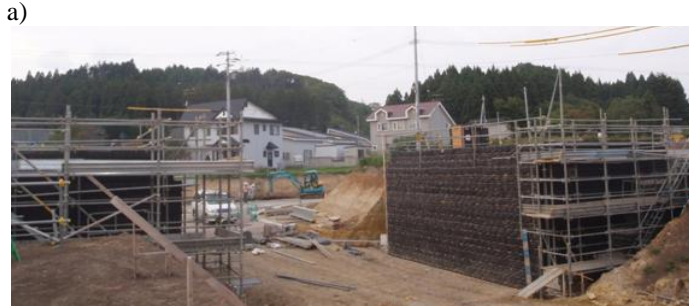
b) Figure 43. First GRS integral bridge, Kikonai at the south end of Hokkaido, for a new bullet train line (11.7 m wide): a) overall structure; and b) abutments under construction, summer 2011 (by the courtesy of Japan Railway Construction, Transport and Technology Agency).
