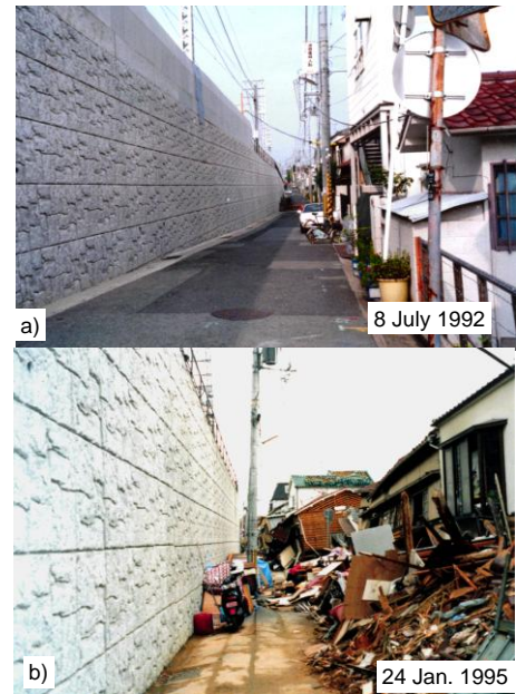
Figure 6. A GRS RW having FHR facing at Tanata, Kobe city; a) immediately after construction; and b) one week after the 1995 Kobe Earthquake (Tatsuoka et al., 1997, 1998).
